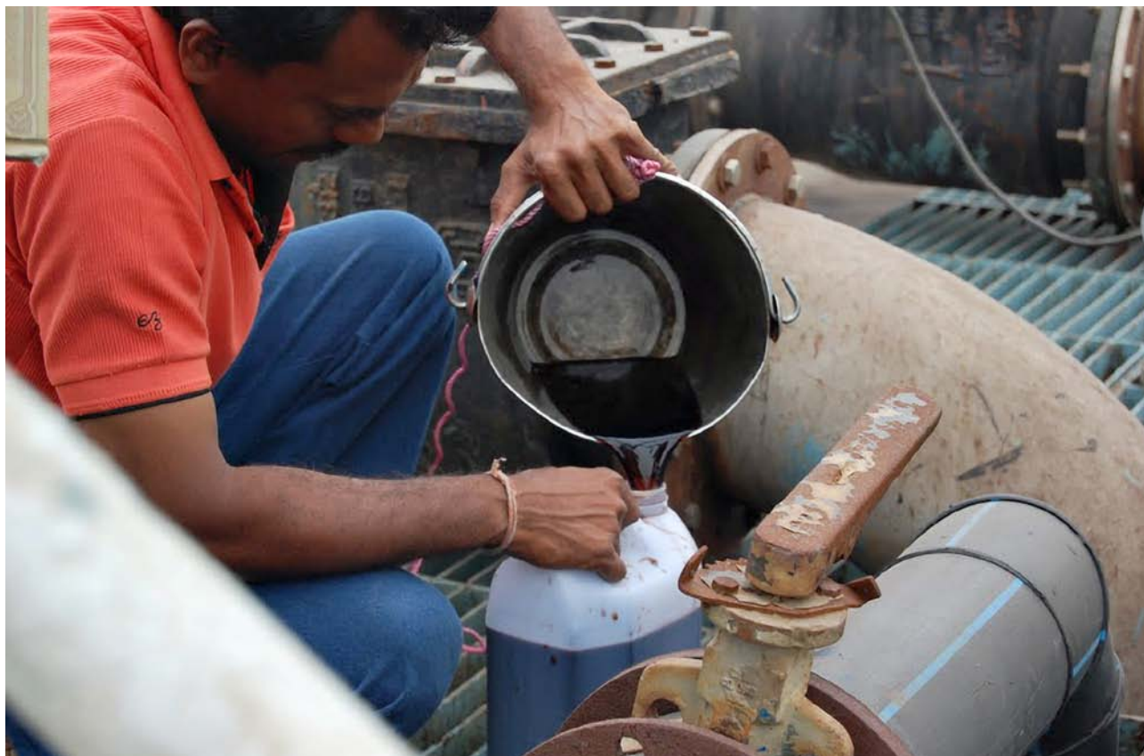
Taking a sample from the outlet of a common effluent treatment plant. Many industrial plants minimally treat their waste effluent before sending it on for further treatment at a common facility. Hence the output of this common facility is very concentrated. Photo: J-PAL
