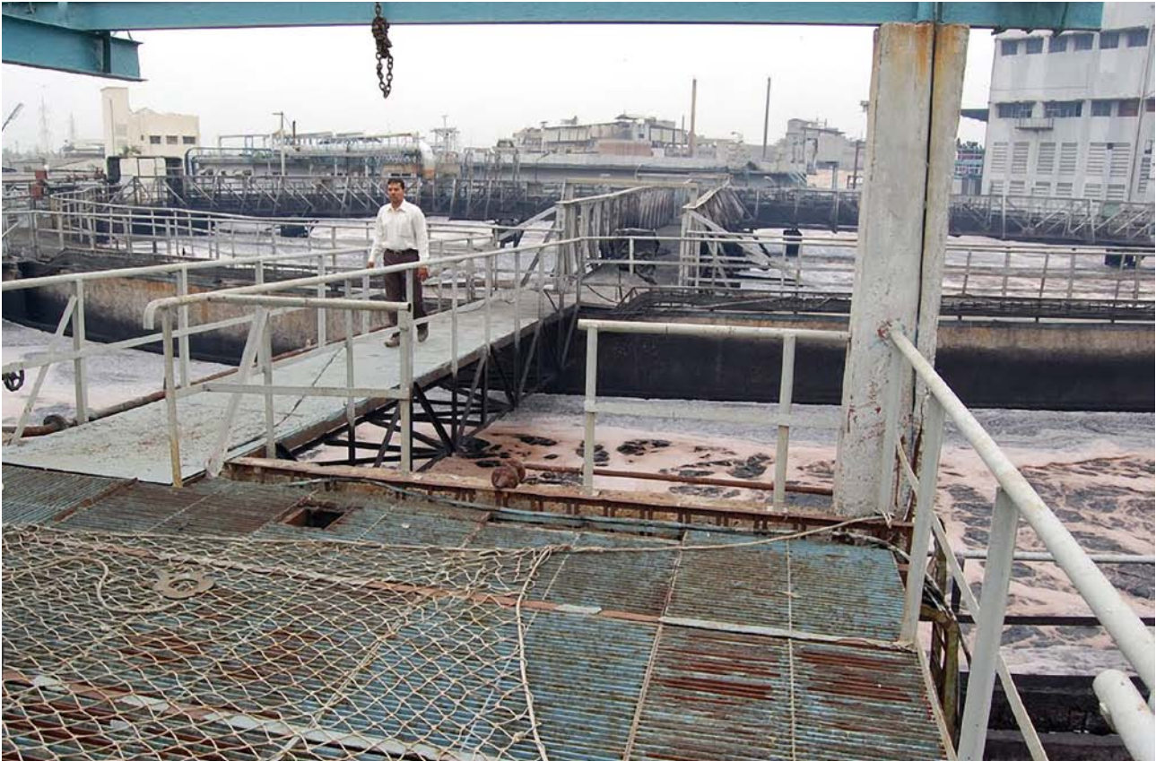
A large tank for biological treatment of waste effluent at a common effluent treatment plant that collects waste effluent from hundreds of small plants. Photo: J-PAL
